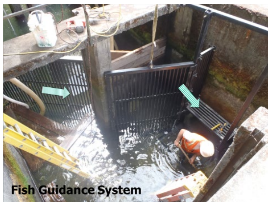
Lower Bennett Weirs (camera installs where worker is located)
